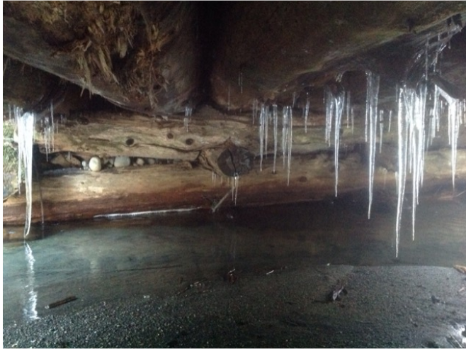
Left Bank Abutment when facing downstream
