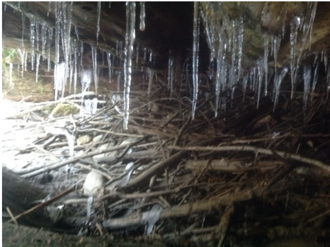
Right Bank Abutment when facing downstream
